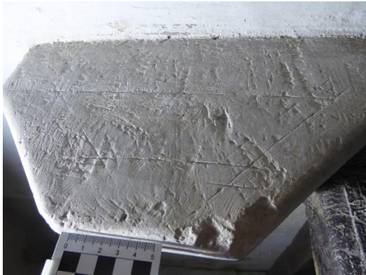
23 North chapel, east wall. Corbel with marking out lines
