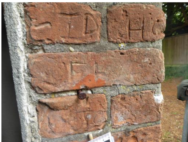
11 South porch doorway, east side. Various initials
