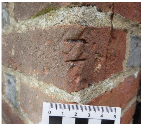
8 Tower, north doorway, east side. Crosses
