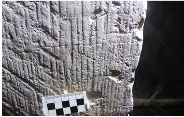
22 North chapel. Arrow shape and marking out lines on west side of doorway
