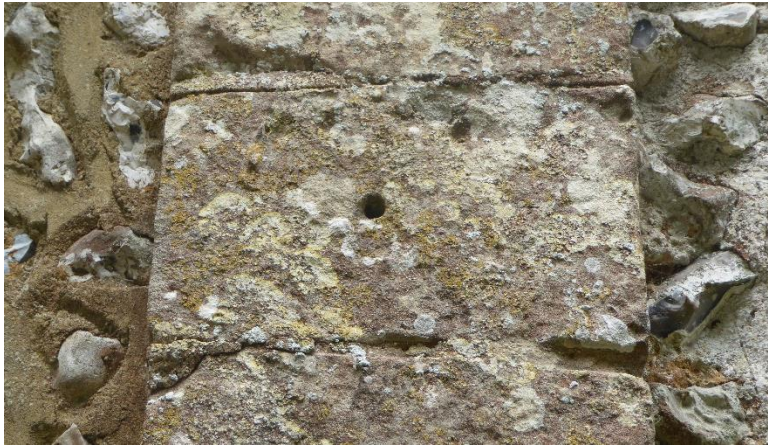
18 South wall. Pilaster strip with block containing hole.
