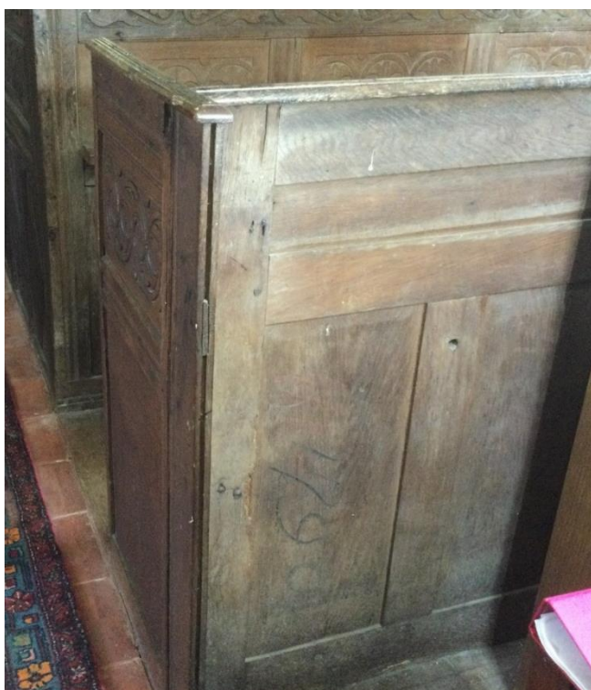
28 Back of box pew next to rood stairs. Painted date 1790
