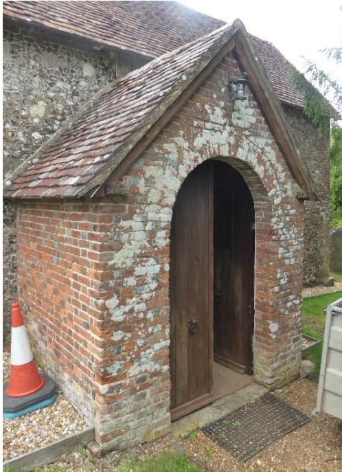
9 The south porch
