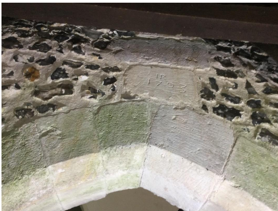
10 South doorway. IR 1703
